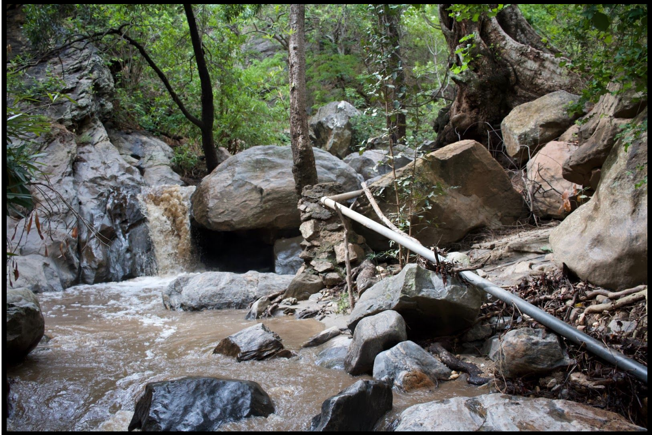
Figure 3.2.3: The government water source and a portion of piping (James Trebesch, January 2018)
