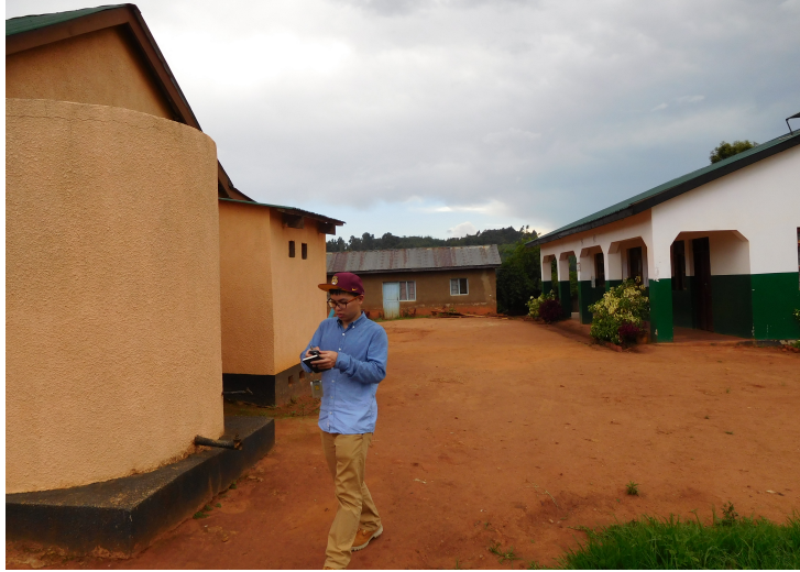
Figure 7 – Proposed site for new tank at the dispensary. Show on the left is the permanent tank that will act as the base for the new tank. The building on the left is to be plumbed during Phase I, and the building to the right is to be plumbed during Phase II.
