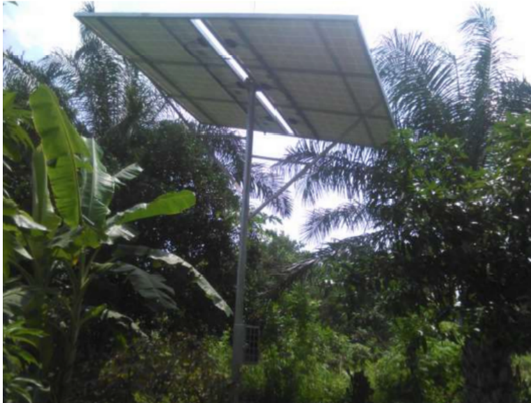
Figure 9 –The Solar Panel Assembly
