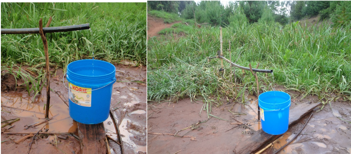
Figures 12: Photographs of the outlet of the Sajeni pipeline in January 2014.
