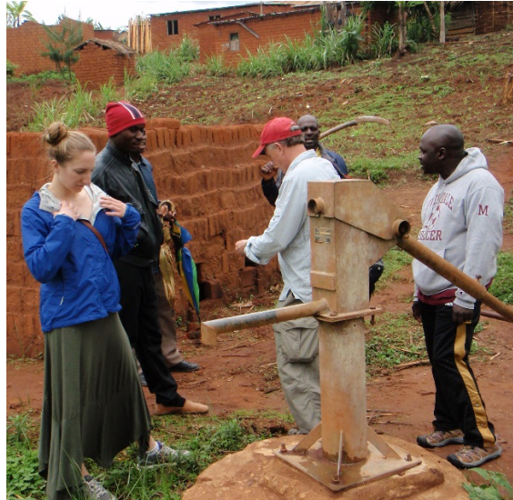
Figures 9: This hand dug well in the village of Kising'a is about 8 m deep and is no longer in working condition. This well was originally intended to serve the primary school [see location (4) in Figure 4].
