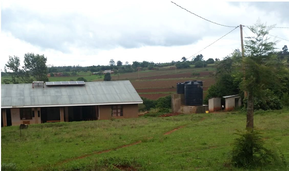
Figure 2.2 Dispensary System. The 2,000 and 10,000 L tanks are seen at right. The solar panel on the roof of the dispensary could be replaced by nearby power lines.
