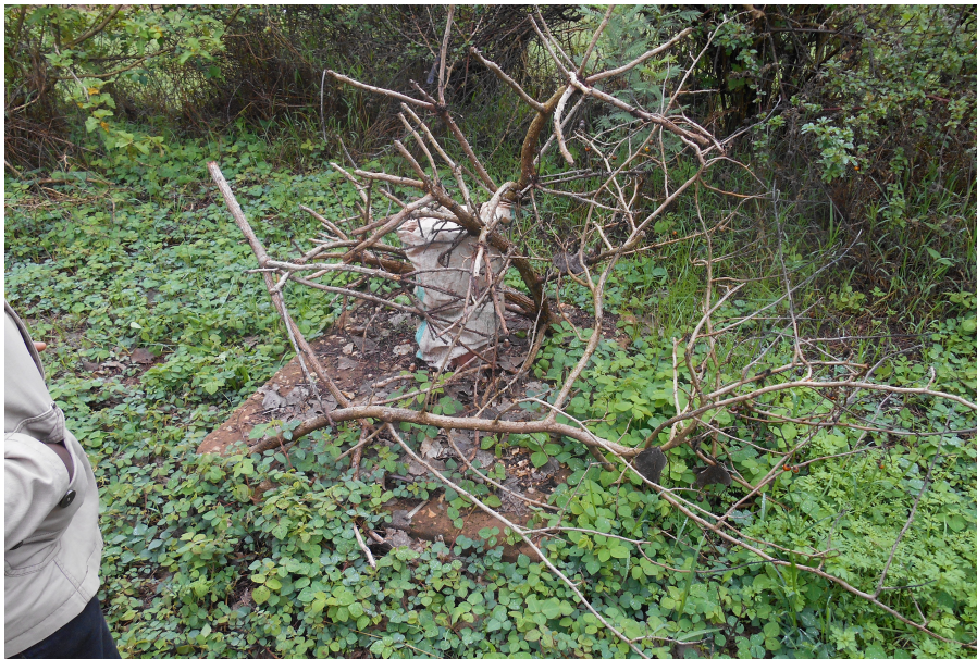
Figure 2.7. East Hand Pump Well (Broken) The borehole has been covered and abandoned until the village decides to repair.
