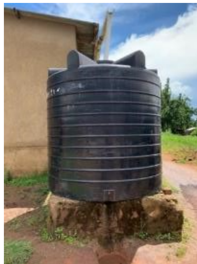
Figure 3.6 | Water Catchment System at Dispensary.
