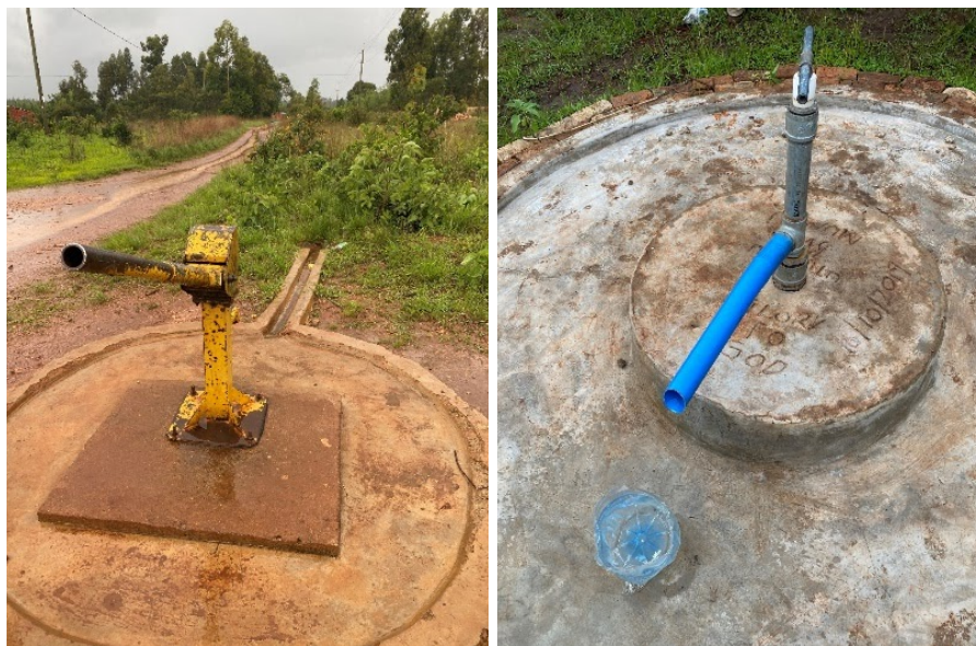
Figure 3.5 and 3.6: Hydraulic hand pump on borehole and hand pump on a hand dug well
