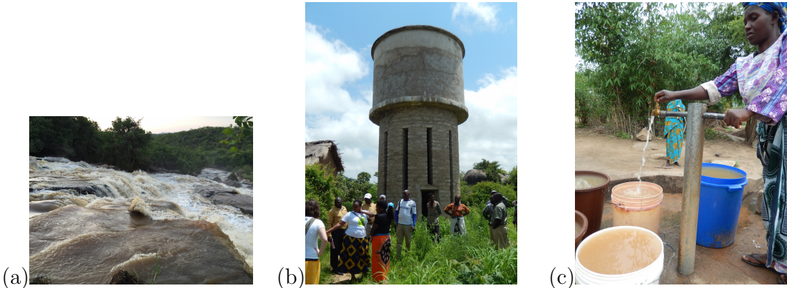
Figure 2: The components of the existing pump system supplying water to Mlangali subvillage consists of (a) river water pumped to a (b) 45,000 L concrete tank where it is then gravity fed to (c) four spigots spanning the length of the subvillage
