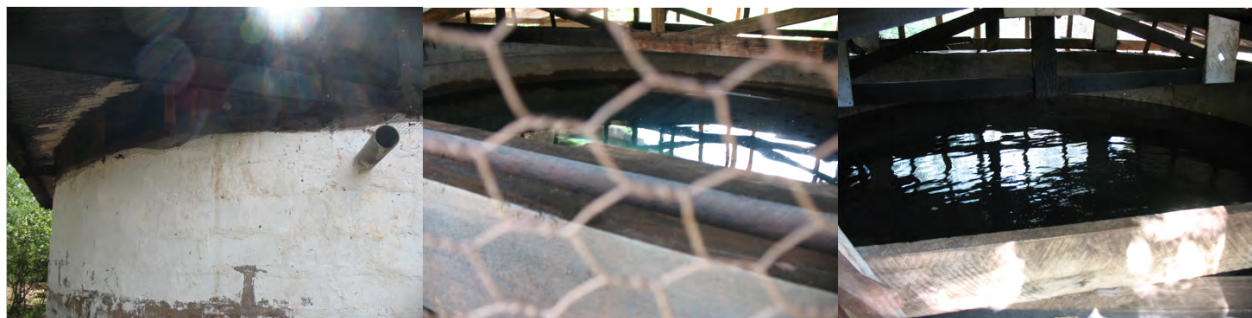
Figure 8: Cisterns at the top of the hill. Left: largest cistern; middle: largest cistern; right: lower cistern.
