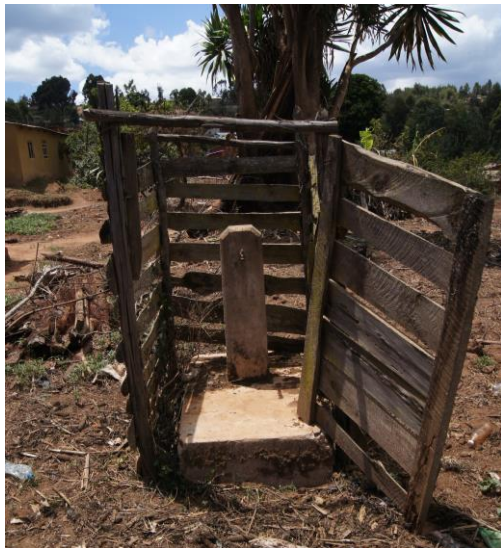
Figure 1.2.4 Distribution Taps in Manyigi. The older distribution taps (a) in Manyigi never were able to deliver water. The newer taps (b) were never connected to a water source.
