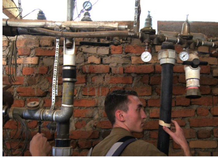
Figure 1.2.2 Water Distribution System in South Mwatasi. The (a) well has a wooden fence that is locked and monitored by the water committee. Inside the (b) pump house, valves can be adjusted to direct the water to the secondary school. (a) 8^{\circ}16'2.30''\text{S } 35^{\circ}48'58.84''\text{E} . (b) 8^{\circ}16'0.47''\text{S } 35^{\circ}49'1.00''\text{E} .
