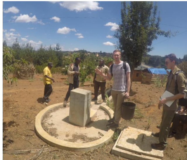
Figure 1.2.4 Distribution Taps in Manyigi. The older distribution taps (a) in Manyigi never were able to deliver water. The newer taps (b) were never connected to a water source.
