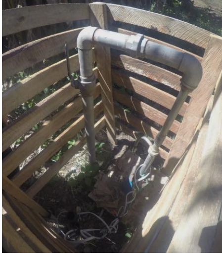
Figure 1.2.2 Water Distribution System in South Mwatasi. The (a) well has a wooden fence that is locked and monitored by the water committee. Inside the (b) pump house, valves can be adjusted to direct the water to the secondary school. (a) 8^{\circ}16'2.30''\text{S } 35^{\circ}48'58.84''\text{E} . (b) 8^{\circ}16'0.47''\text{S } 35^{\circ}49'1.00''\text{E} .
