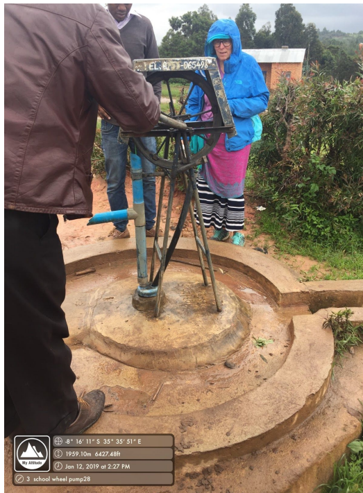
Figure 7: Rope pump dug in 2015 and currently used by students at Mong’a primary school. Well depth is 9.1 m and original water level was 1.5 m. In the wet season this pump fills approximately 15 to 20 buckets at a time and requires 12 hours to refill while in the dry season the pump fills 1 to 2 buckets at a time and requires 24 hours to refill.
