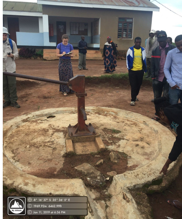
Figure 6: Hand pump near dispensary. Well depth is 36 m and the original water level was 12 m. Ran dry in February 2018.
