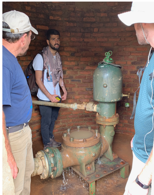
Figure 3.4 Hydraulic Ram Pump
