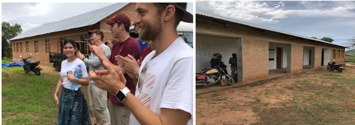
Figure 5.3 The Village Office in Wangama. The roof will be suitable to hold the solar array that will power the pump in the borehole.
