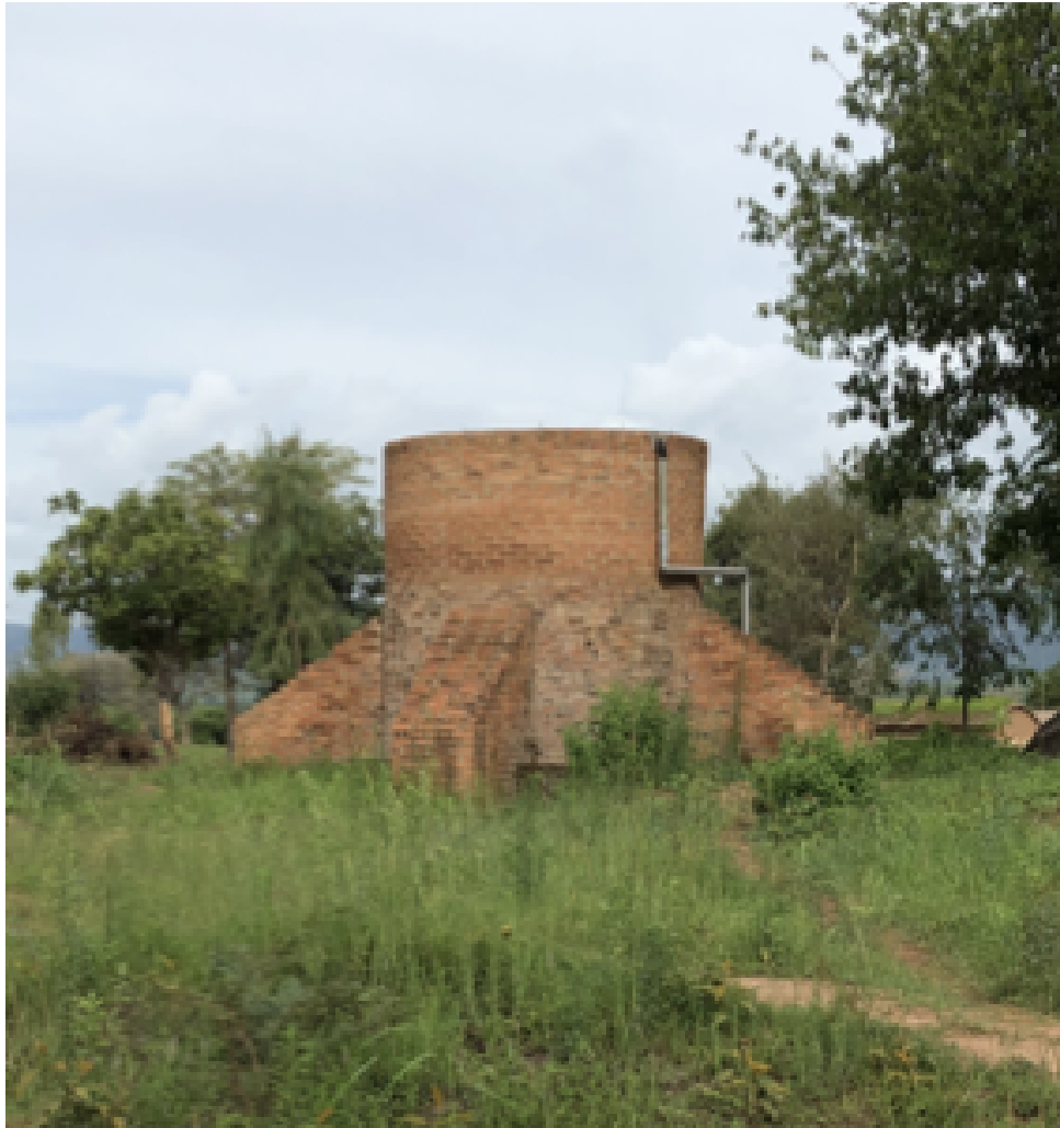
Figure 3.1 The brick storage tank at Village Office with an elevation of 1647.1 meters (5404 feet).
